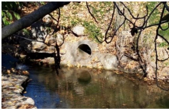
Figura 13: Sobreexidor del Pg. Colomer (41.5268040, 2.0870130)
